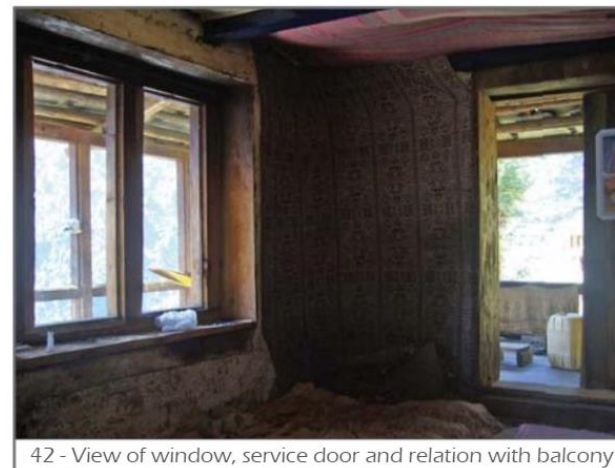
42 - View of window, service door and relation with balcony
